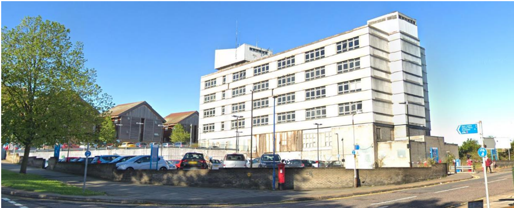
Plate 8: Eastern boundary and M Block from the corner of Bath Street and Clifton Road (facing SW)
